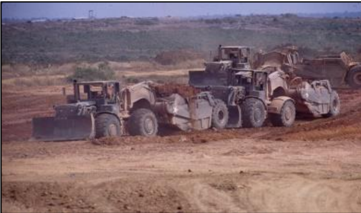
Above is a photo from March, 1972 showing several of them pushing each other through a borrow pit in Bien Hoa RVN. Bulldozers were also employed as pushers in borrow pits.
