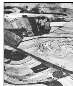
The village of Ouren, Belgium, which contained two bridges over the Our behind the 112 th Infantry. In the top of the photo the Weiswampach road runs along a tall ridgeline overlooking the town
